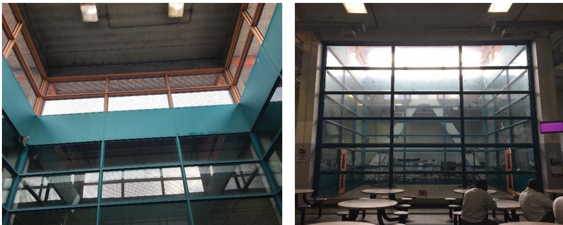
Figure 7. Mesh cages added to glass enclosure inside housing areas to provide “outdoor” recreation for detainees. Observed by OIG at the Essex Facility on July 24, 2018. Source: OIG
